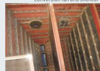
引风系统变频风机和消音器 Air induction system frequency conversion fan and silencer
